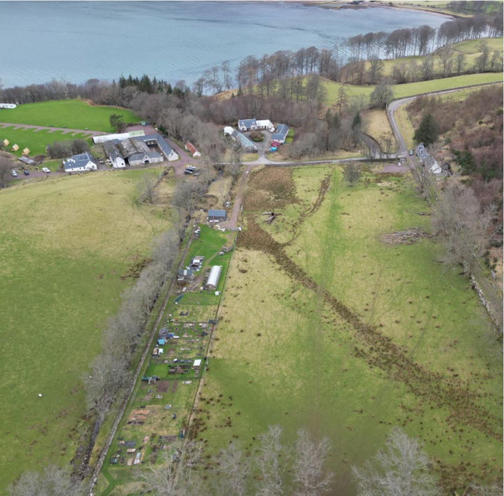
Aerial Photo Showing Site
